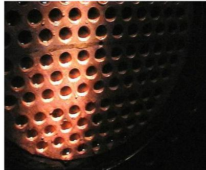
Water scale on any heat transfer surface reduces the effectiveness of that heat transfer. This results in reduced equipment efficiency while increasing energy consumption, increasing costs and even increasing plant downtime. Often this "buildup" problem is either ignored or relegated to "fixing it at the last minute or upon mechanical failure" status because of downtime costs. This is historically based on the premise that to descale takes a great deal of time.
